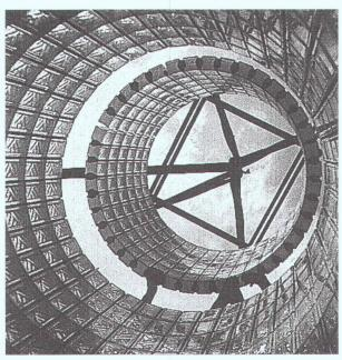
BRIQUES DE VERRE PRÉFABRICATION MAÇONNAGE SUR CHANTIER
