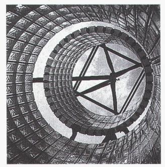
BRIQUES DE VERRE PRÉFABRICATION MAÇONNAGE SUR CHANTIER
