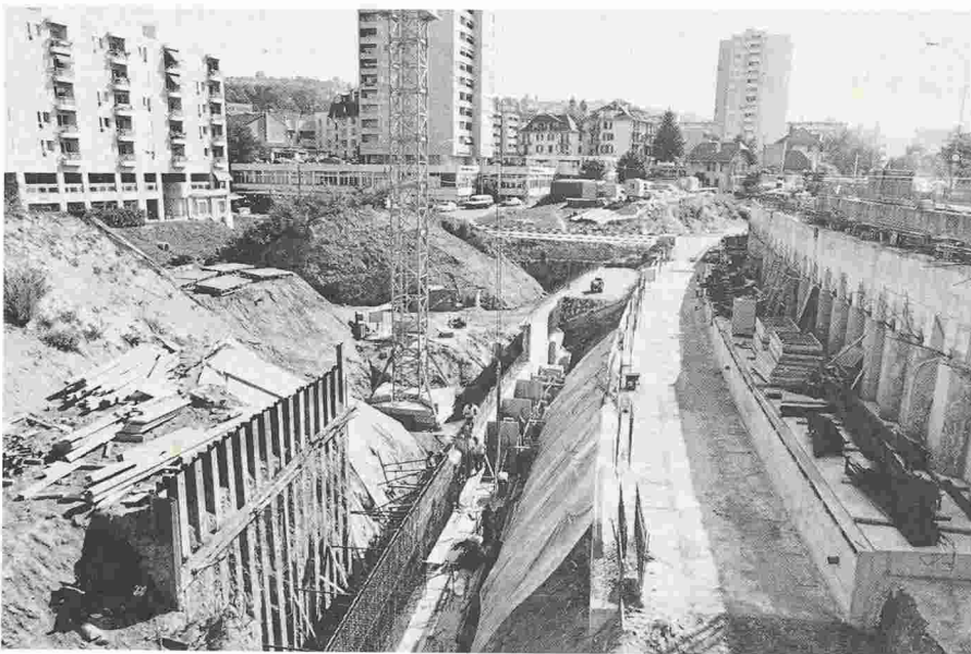
Fig. 16. – Station de Malley.
