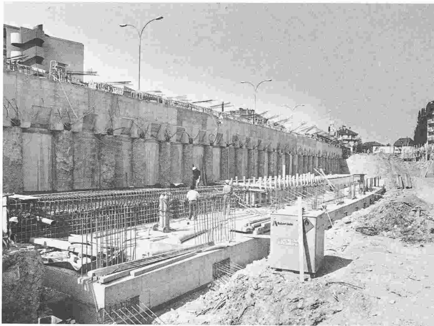
Fig. 15. – Station de Malley.
