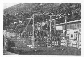
Fig. 7. — Vissoie, 1957. l = 7 m; H = 3 t;  $k_2 = 36 \text{ kg/m}^2$ ; T = 65 kV
