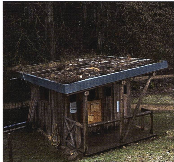
Figure 2. General view of the Soil House from the north-west on 9 January 2022. Note the “refrigerator” effect of the frozen ground on the roof, which keeps snow in place longer than in the surrounding meadow and forest.
