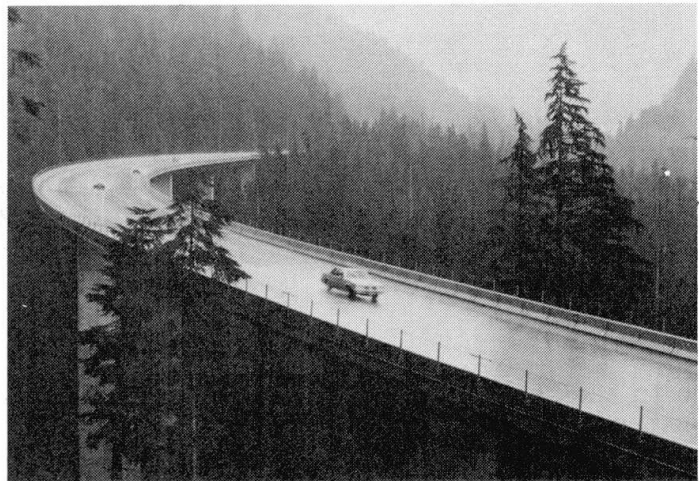
Fig. 13 Denny Creek Bridge Washington
