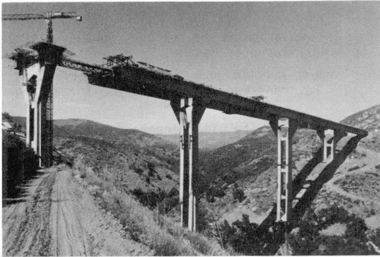
Fig. 3 Pine Valley Creek Bridge California
