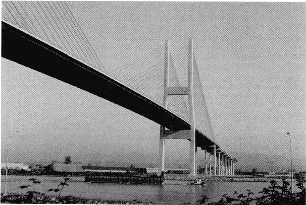
Figure 5. Alex Fraser Bridge.
