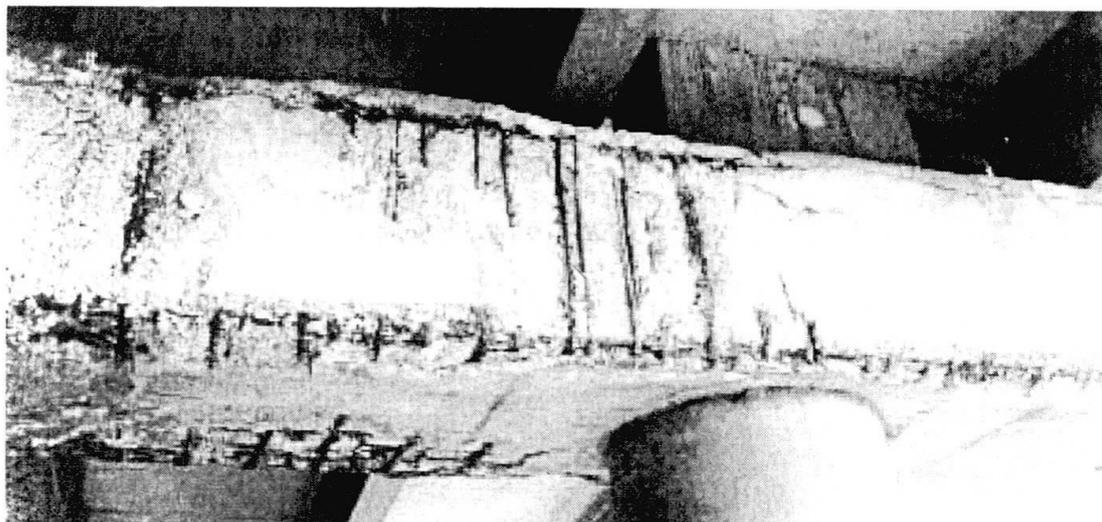
*Fig. 1 An Example of a Deteriorated Crossbeam*
