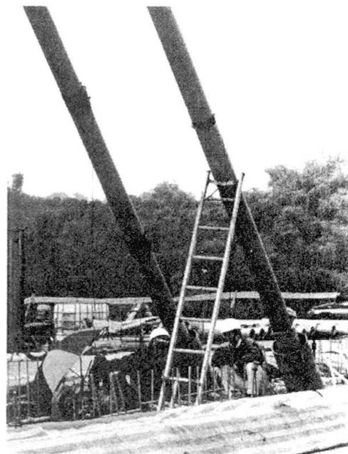
Fig. 3 Cable forces checked by ambient vibration method
