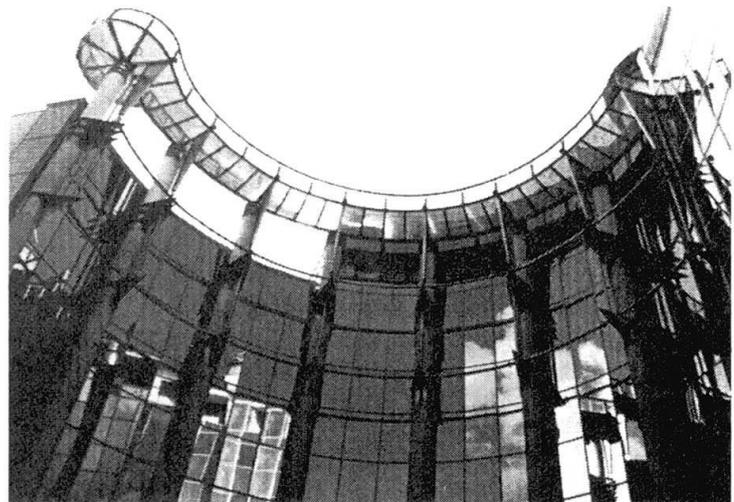
*Fig. 2 Backyard facade - curved roof footbridge with transparent grill footpath*
