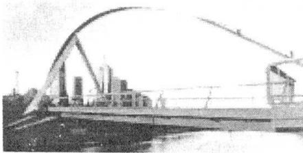
An example on an arch bridge designed without considering the principles outlined above, is shown in Fig.2. Here the load from the bridge deck is transferred at one point so the correct form of the arch would have been two straight members leading directly to the supporting points. However, the designer apparently found a curved arch to look nicer so this form was chosen despite the consequences regarding material consumption.
