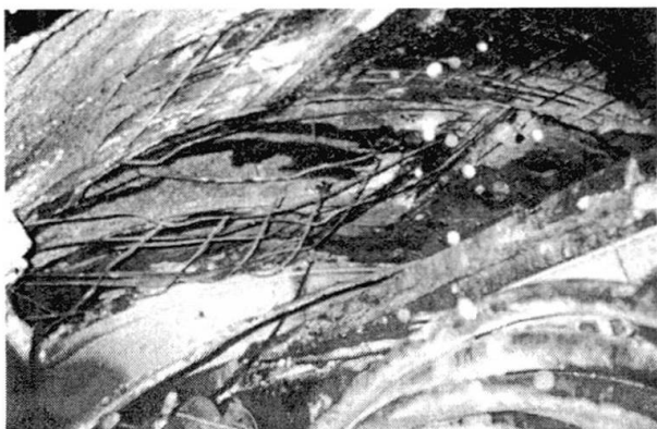
Great Belt Tunnel after a fire during construction.
