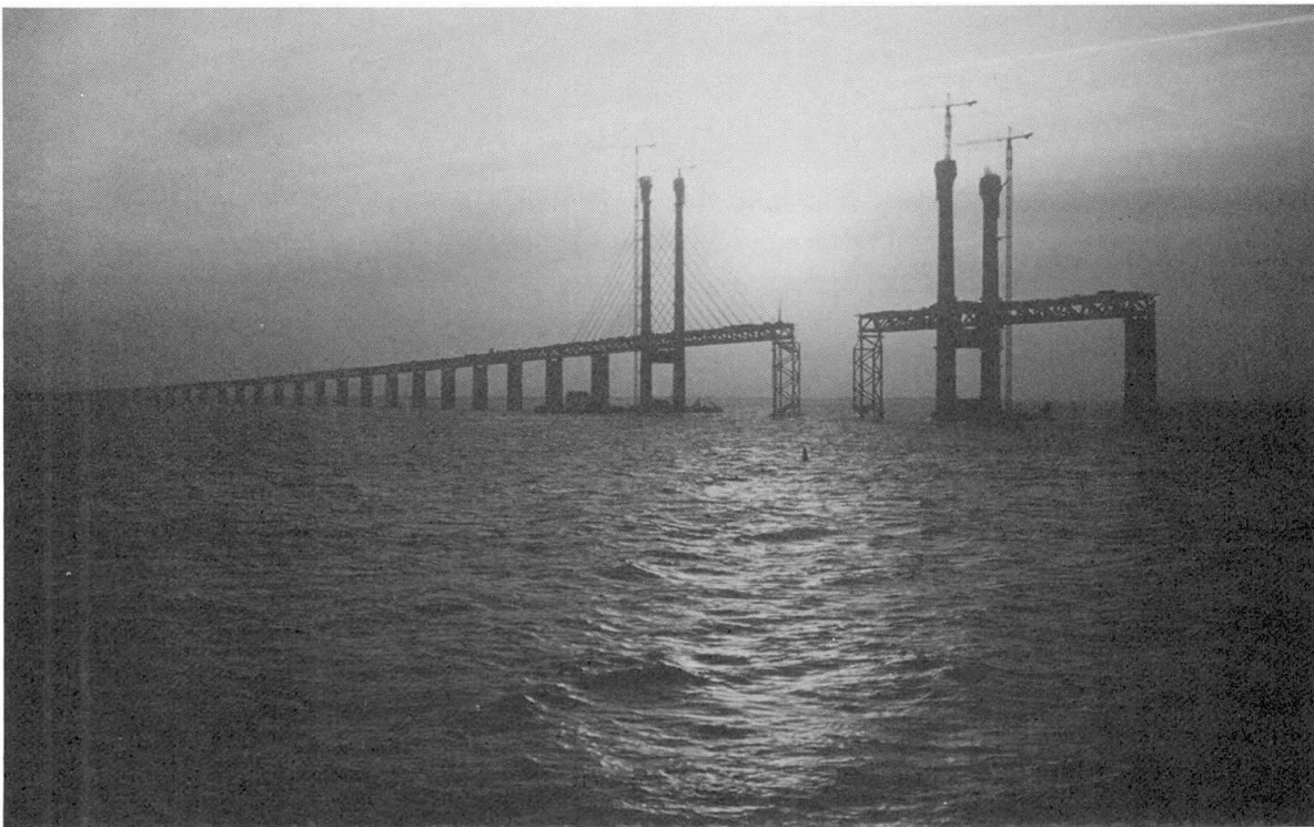
The 490m main span is nearing completion
