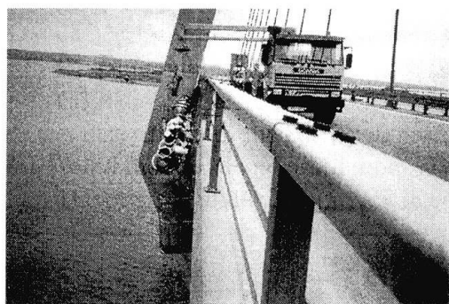
Figure 3 Access equipment, Bucket snooper boom and Skyclimber platform
