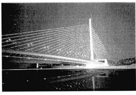
The main span of the bridge over the river is 162 m long, in continuity with a short 31 m long span above the left embankment and a very short 12 m long span between the pylon and the balancing abutment. This abutment is 122 m long and is the first part of a tunnel that goes on under the railway junction.
