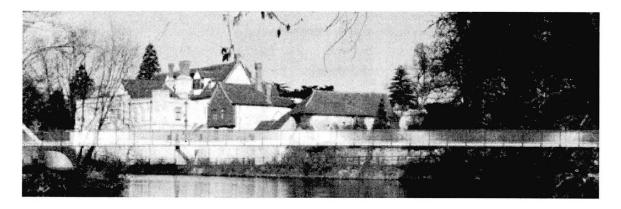
The bridge spans both the river and the adjacent floodplain on one side, and is 90 metres long overall. The sculpted form of the central concrete support cuts the floodwaters like the bow of a boat and carries a stair on its back. This "cutwater" pier stands on one bank of the river and supports twin skeletal steel masts inclined outwards in a wide V shape from which galvanised steel locked coil ropes support the lightweight deck.
