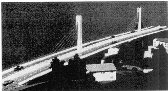
For the case of Fig. 1, the use of stays allowed to keep the same type of cross section of the typical spans (a voided slab deck) at the severe end span 61m long. For the viaduct in Fig. 2, it was important to use an axial stay-cable deck with a slender cross section. A triangular type box girder section was adopted and wind tunnel tests have shown an excellent aerodynamic stability.
