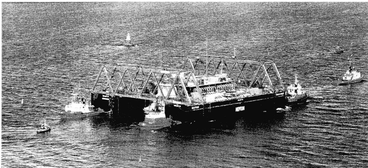
West Caisson during Towing
