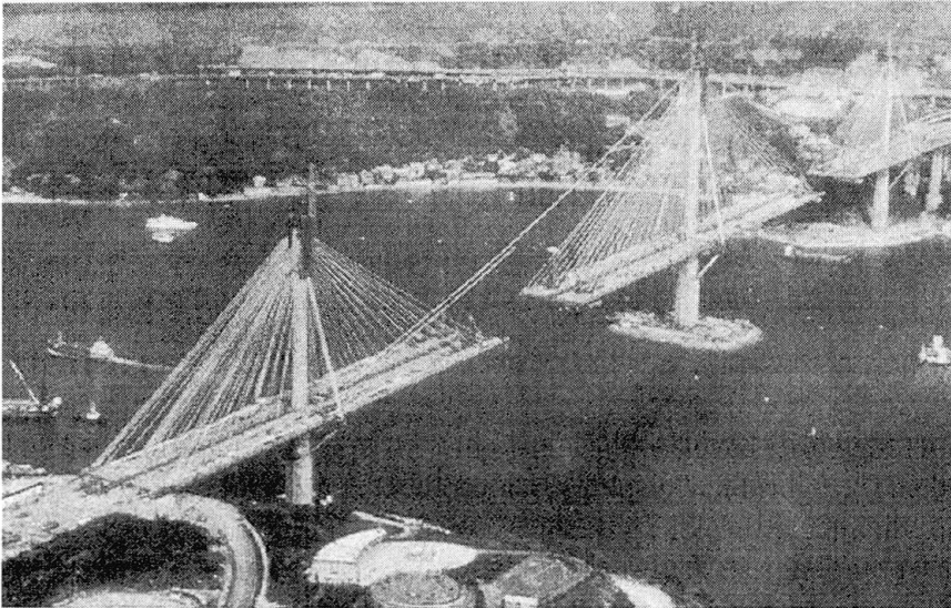
Fig. 1: Ting Kau Cable Stayed Bridge Erection
