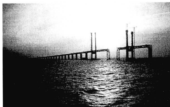
The cable-stayed bridge nearing completion
