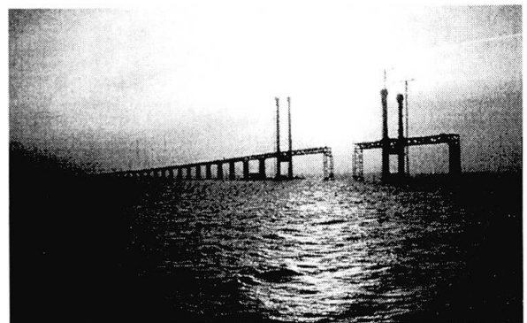
The cable-stayed bridge nearing completion
