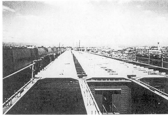
Fig.7 Setting of Bottom form on girders
