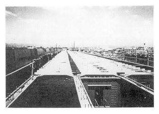
Fig.6 Erection of Bottom form
