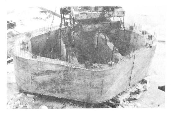
Fig. 3. Ice protective shell
