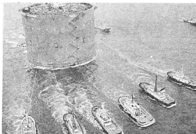
Photo-1 Laying-down Caisson Method (Towing Steel Caisson of 2P)
