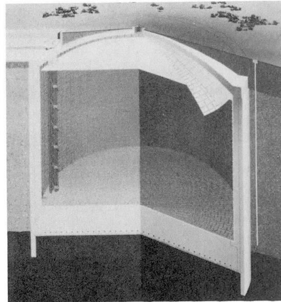
Fig. 1 General view of 200,000 kl LNG underground tank
