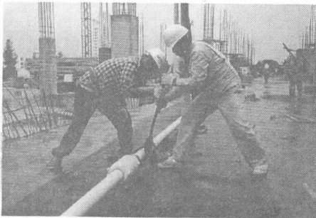
Photo 5: Assembly of tie rod
