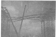
Photo 4: Installation of main truss
