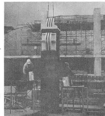
Photo 2: Assembly of embedded column
