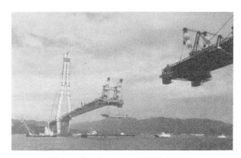
Photo. 2 Erection of Steel Girder
