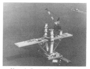
Photo. 1 Erection by Tower Crane
