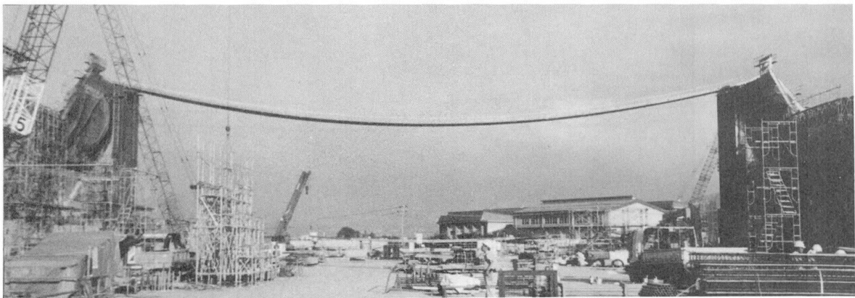
Photo. 5 Overview of the Actual Lift-Up State
