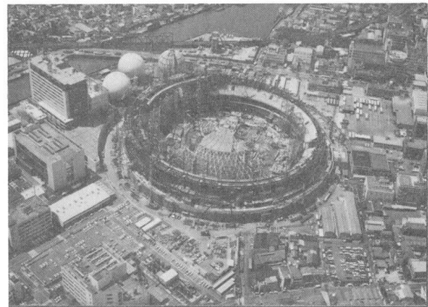
Erection of roof truss on the ground level
