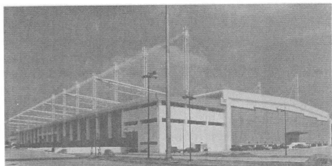
Photo 1: Overall view of building
