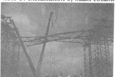
Photo 4: Installation of main truss
