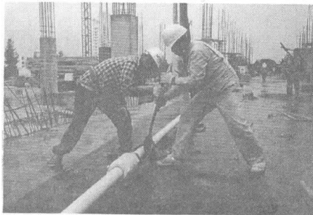
Photo 5: Assembly of tie rod
