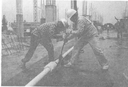
Photo 5: Assembly of tie rod
