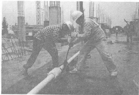
Photo 5: Assembly of tie rod
