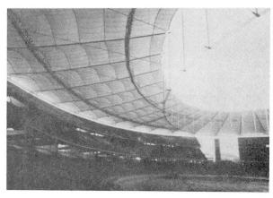
Fig. 15 Lightweight Roof structures for the Outdoor Stadium Kuala Lumpur, Malaysia. This cable membrane roof covers 100,000 seats and with 38,500 m² roof area has become the largest stadium of the world.
