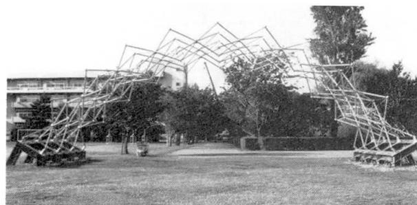
Fig.25 Test building of Tensegric Truss Arch (1997)
