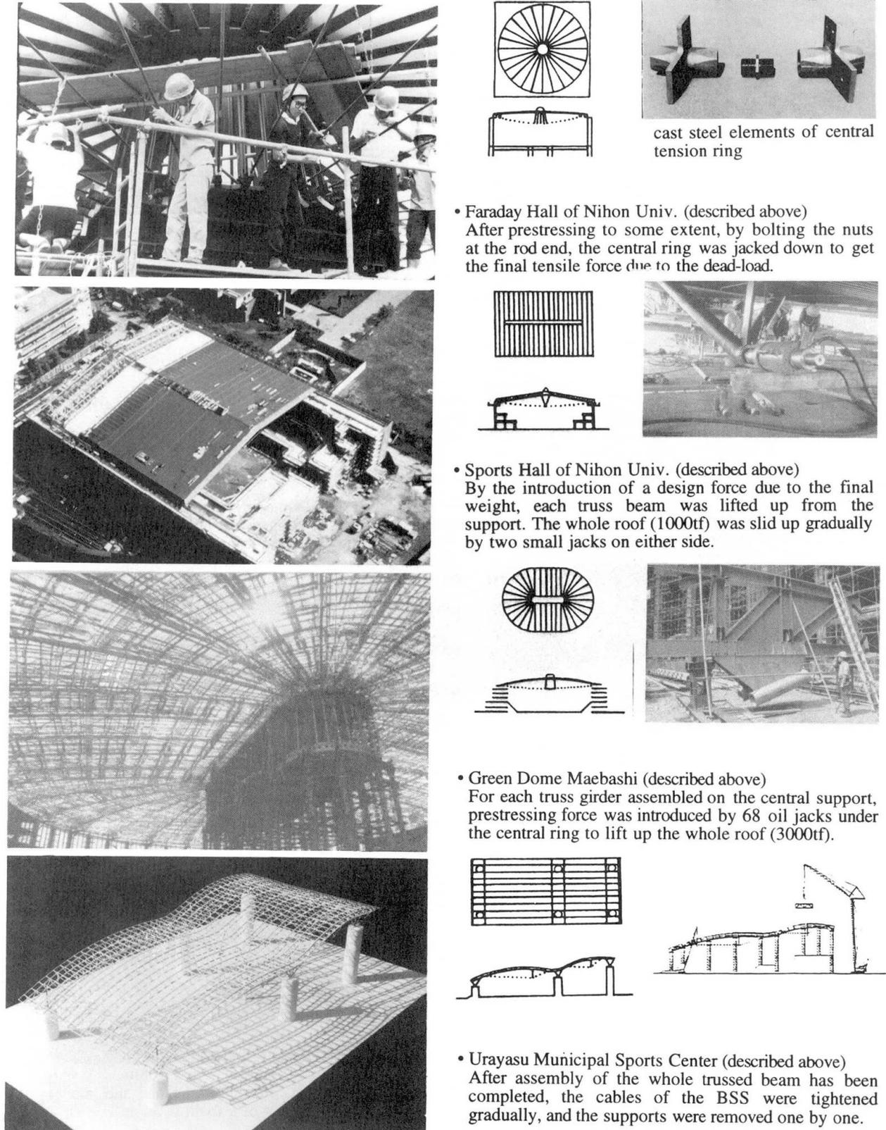
Fig.14 The example of prestressing and construction method (1)
