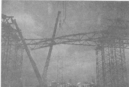
Photo 4: Installation of main truss
