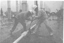
Photo 5: Assembly of tie rod
