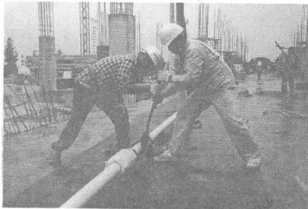
Photo 5: Assembly of tie rod
