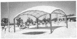
• System truss with screw bolts joint Fig.17 EP dome with four columns (1997)
