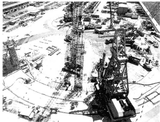
Photo 1 Work of Underground Slurry Wall
