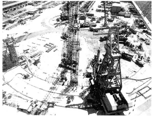
Photo 1 Work of Underground Slurry Wall
