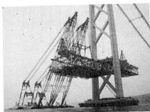
Photo. 4 Large-Block truss girder erection
