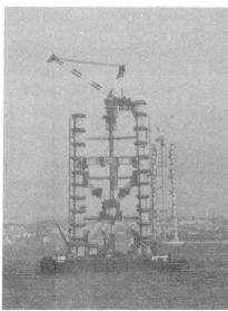
Photo. 1 Erection by Climbing
