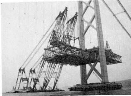
Photo. 4 Large-Block truss girder erection
