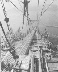
Photo.3 Strand erection by hauling system
