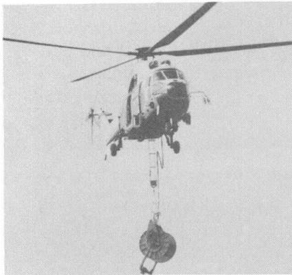
Photo.2 Carrying a pilot rope by helicopter
