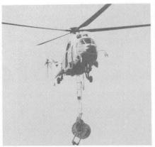
Photo.2 Carrying a pilot rope by helicopter
