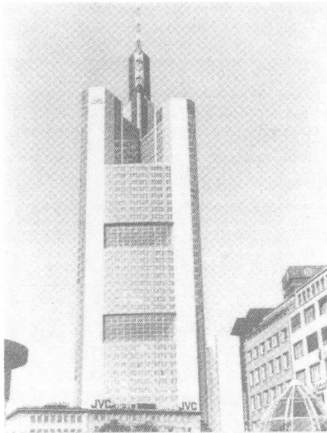
Fig. 1: Eastern elevation of the new Commerzbank-Building
