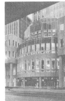
26 The base of North West Tower
