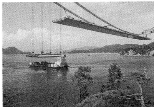
Fig. 4 View of the girder erection
