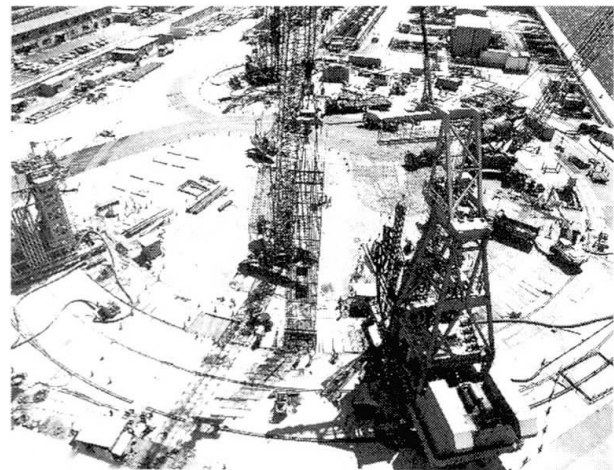
Photo 1 Work of Underground Slurry Wall
