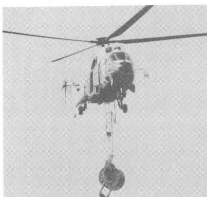
Photo.2 Carrying a pilot rope by helicopter
