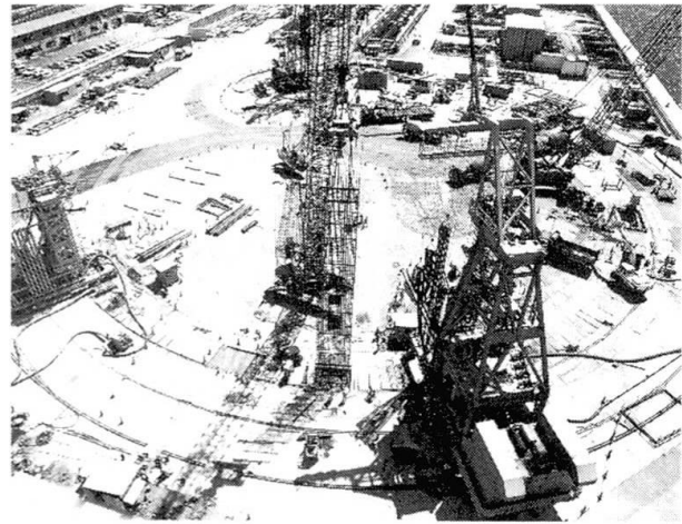
Photo 1 Work of Underground Slurry Wall
