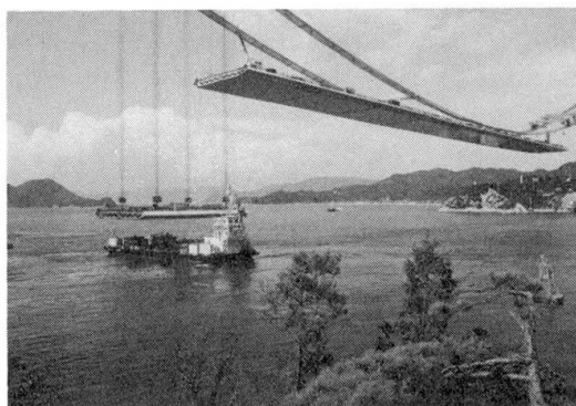
Fig.4 View of the girder erection
