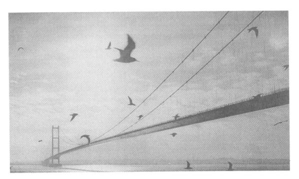
Figure 1 - Humber Bridge showing slender box and inclined hangers
