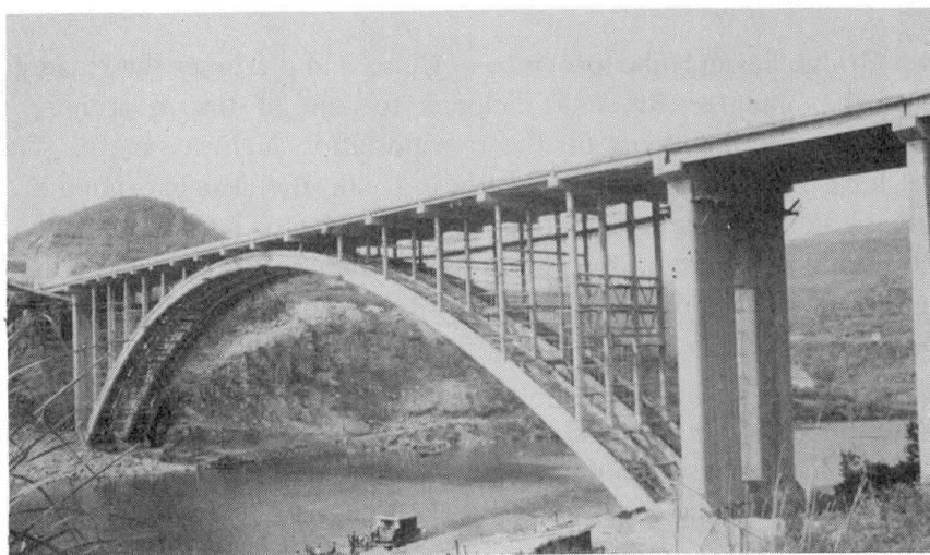
Fig.2 The Huangbai River Bridge
