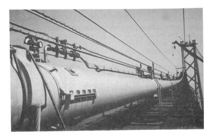
Photo 1 Dry air injection (exhaust) cover
