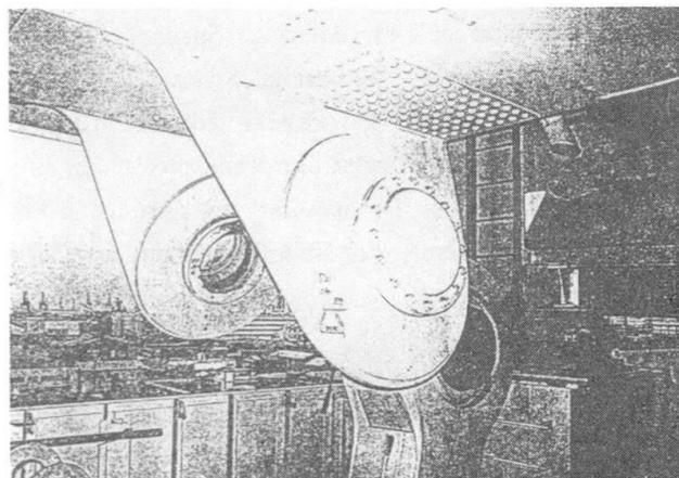
**Fig. 2 Higashi-Kobe Bridge damage of pendel type bearing**
