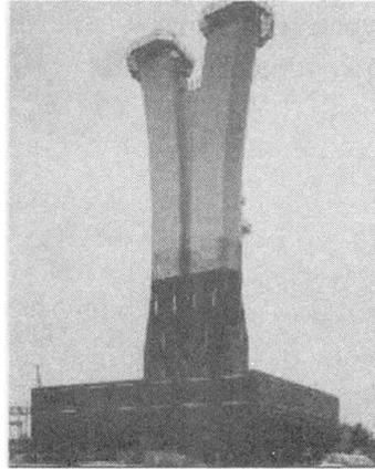
Fig. 2 Steel pier of Trans-Tokyo Bay Bridge
