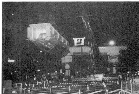
Photo. 3 Erection of Girder and Deck
