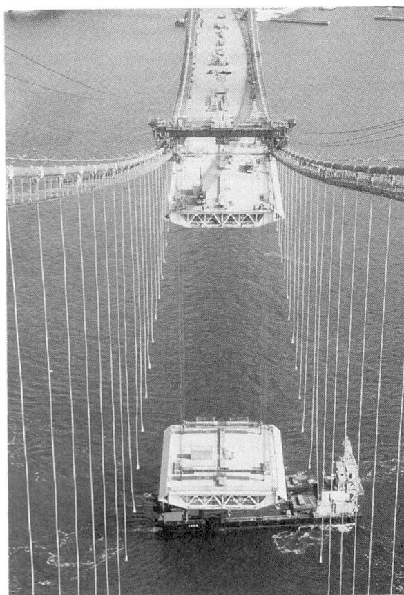
Photo 4 The Large-Block Girder Erection by Dynamic Positioning System
