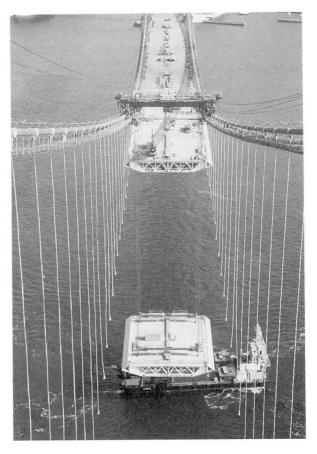
Photo 4 The Large-Block Girder Erection by Dynamic Positioning System
