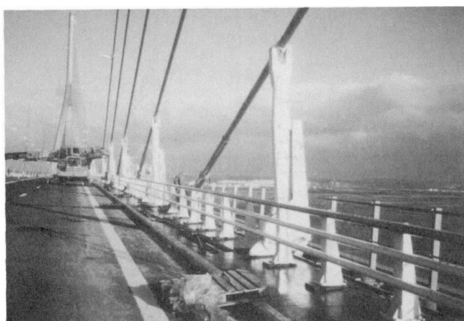
Normandie Bridge : Damping ropes and hydraulic dampers
