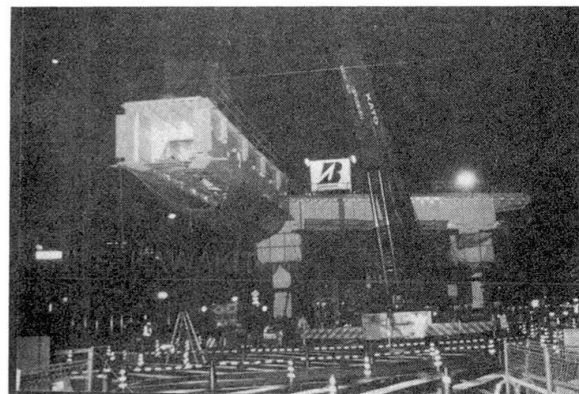
Photo. 3 Erection of Girder and Deck
