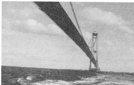
Fig. 5 - 6 - Installing suspension bridge sections
