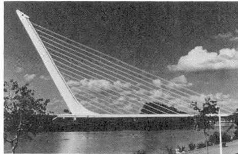
*Fig. 7 The Alamillo Bridge in Sevilla. The combination of a heavy, leaning concrete pylon and a lightweight bridge deck balances in a clever way the dead load but under traffic load large moments will be induced in the pylon and its foundation*
