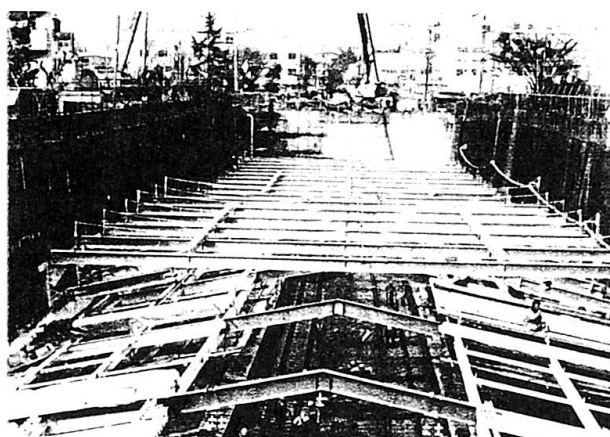
Photo 5 Installation of Struts
