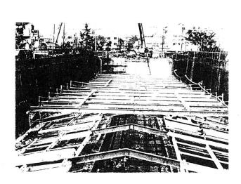
Photo 5 Installation of Struts
