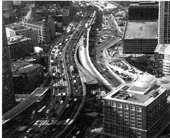
View 2 Looking along the I-93 alignment north. View shows new temporary ramp and construction below existing artery.
