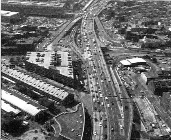
View 1 Looking along the I-93 alignment north. Callahan and Sumner Tunnel portals on the right.
