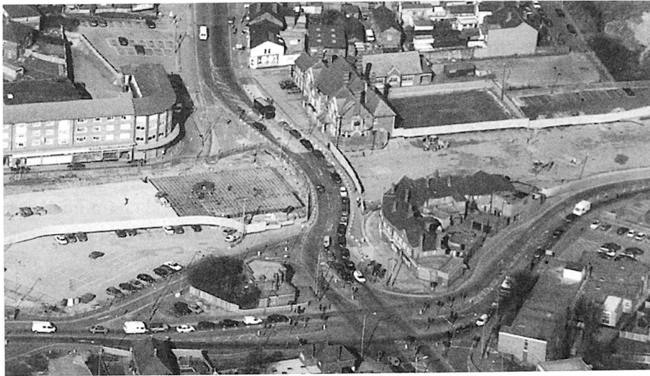
Figure 2: Road diversion during tunnel construction
