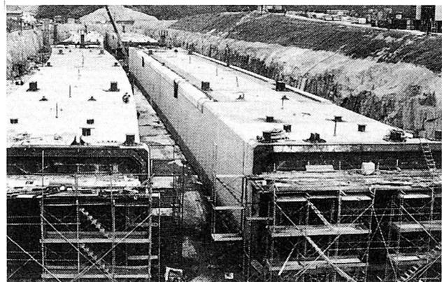
*Fig 3 Tunnel Units under Construction*
